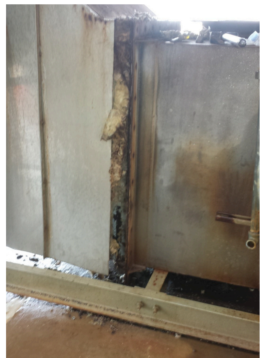
BEFORE: Connection at exhaust stack
