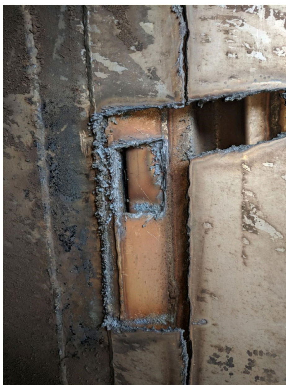
BEFORE: Expansion joint - 3 layers of liners
