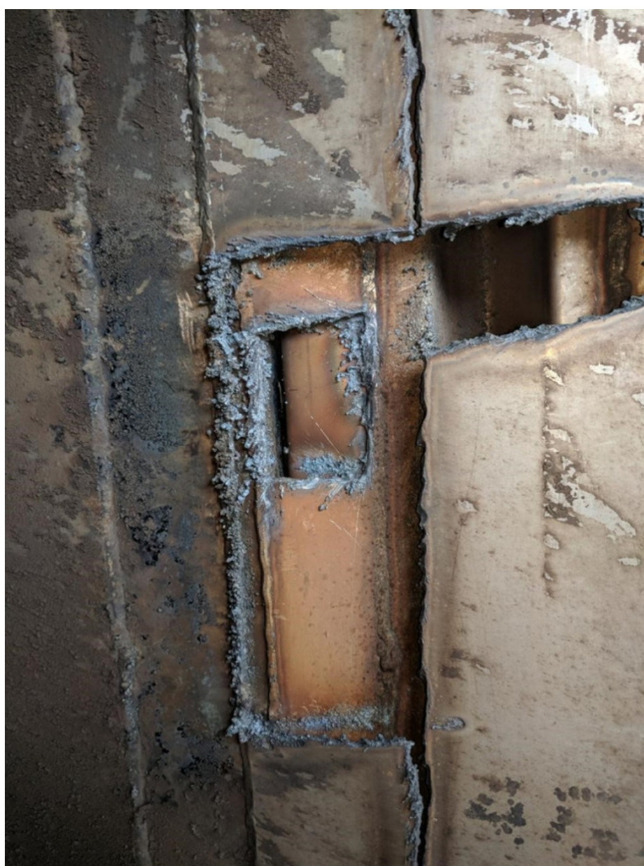
BEFORE: Expansion joint - 3 layers of liners
